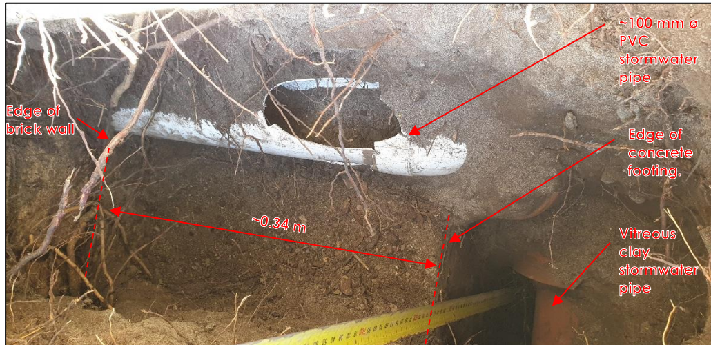
Photo 2: Concrete footing exposed in test pit TP101.
